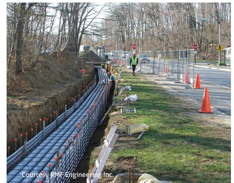
Many campus electrical distribution systems are reaching the end of their useful life.
