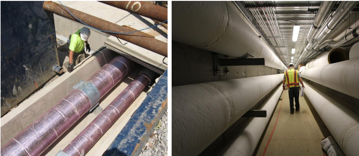
Figure 7 – Thermal Piping in Trench/Coffer and Walkable Tunnel
